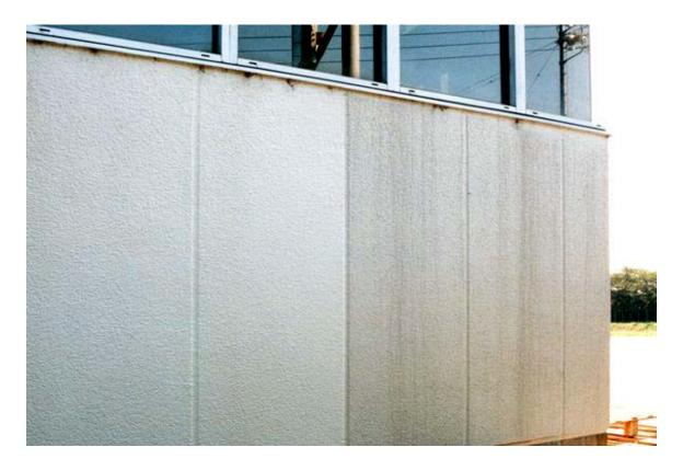
The treated left side of this exterior wall has retained its original clean appearance. The untreated right side of the wall is discolored with grime. The photocatalyst was applied August, 1999 and the photograph was taken September, 2004. The treated left side will continue to remain clean because contaminants are continuously oxidized on the surface by the light-activated photocatalyst. Dirt and oils are washed off with each rainstorm.
