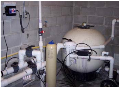
Savastat P-160 is strapped on pipe between the pump and filter using a 110V power supply.
