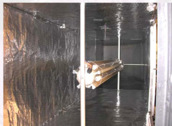
Figure 2-2. Device installed inside the test rig. There are 5 lamps. A reflective surface was placed in the duct.
