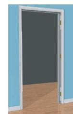
3. Slide Jamb Shield over jamb. Pre-drill holes into stud and secure piece with screws (included).
