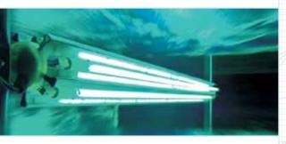
Installing parallel to the air-stream increases dwell time (contact time) with air
