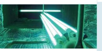
Severe chemical and odor applications: a single Multi-split lamp working in conjunction with the UV bio-wall is installed up-stream
