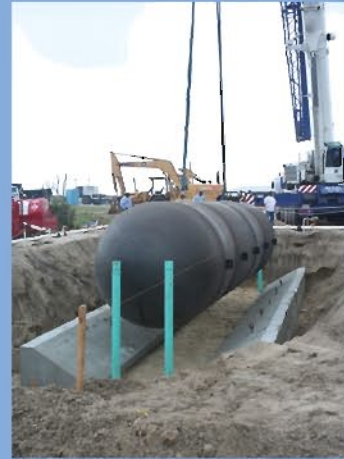
Underground Tank Installation
