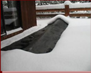
Concrete Curing
