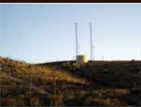
Artesian Well with Water Storage Tanks
