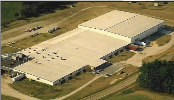
208,650 SF Manufacturing/Warehouse, Red Springs, NC RESERVE PRICE: $485,000
