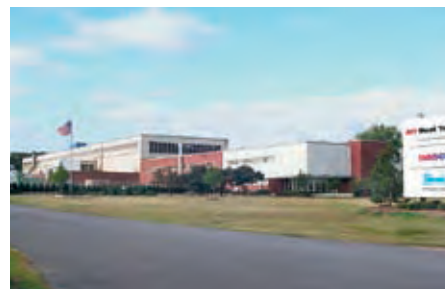
API Basco facilities
