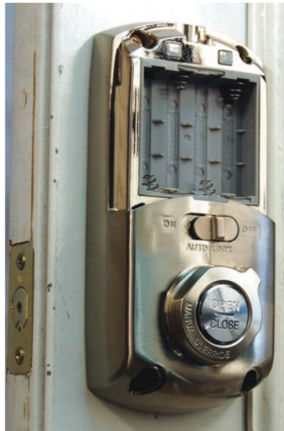
19. The interior unit is held in place with 4 screws.
