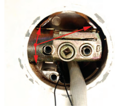
16. With the throwbolt installed, the exterior unit can be slid into place.
