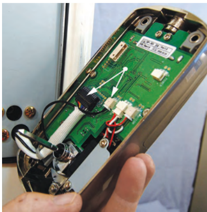
18. Two wire connections are made before installing the interior unit.
