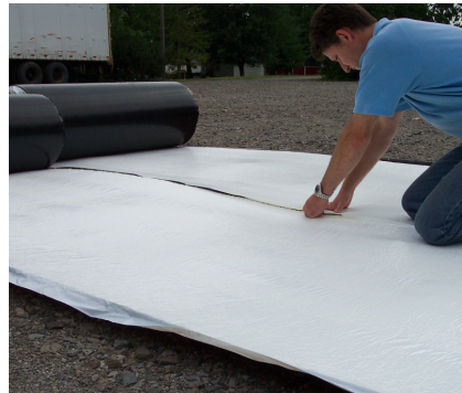
LAY DOWN TUBING / SEAL AROUND OPENINGS
