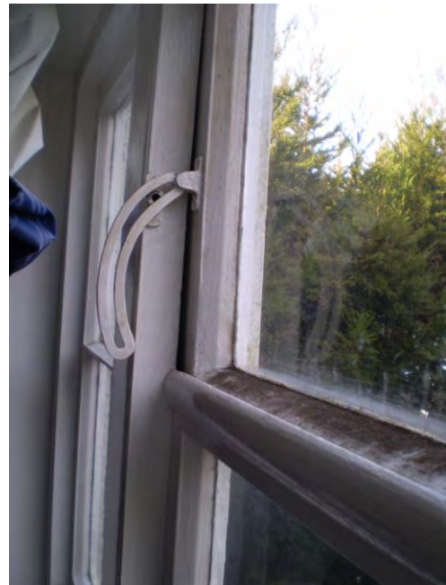
Photos of broken window clasps that do not allow the windows to be closed tightly and blown open when windy. There are also significant gaps around the windows.
