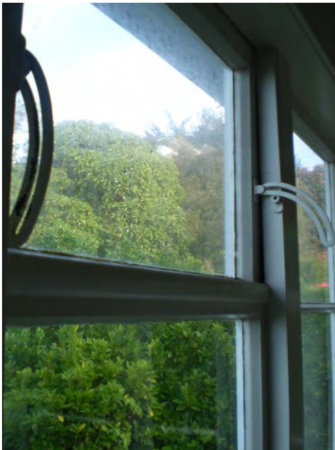
Photos of broken window clasps that do not allow the windows to be closed tightly and blown open when windy. There are also significant gaps around the windows.
