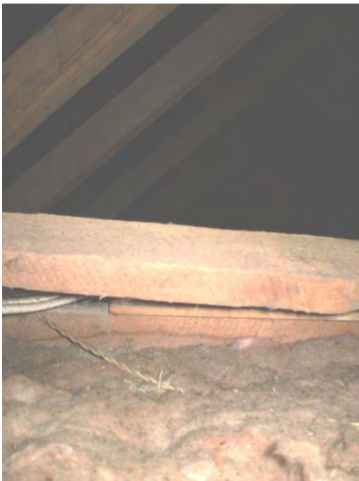
Photo of accessible ceiling space. The existing insulation has been disturbed over the years and has also settled reducing its insulation value.
