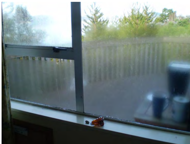
Photo of condensation on the master bedroom windows.
