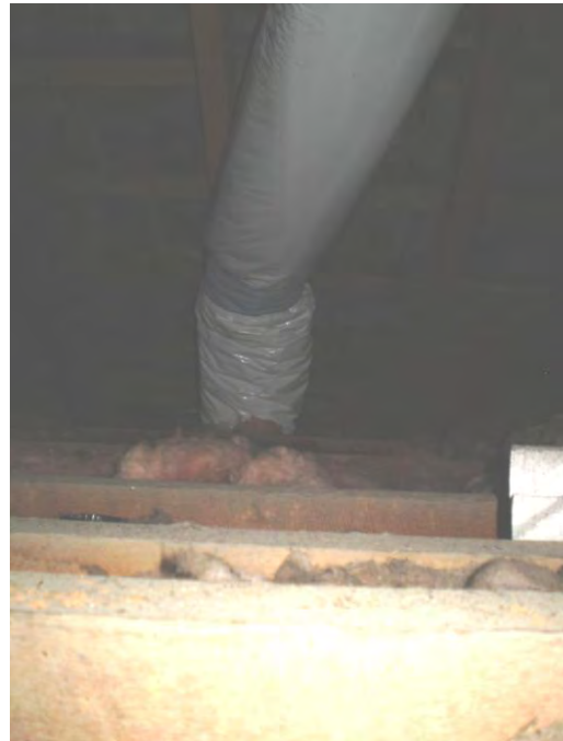
Photo of accessible ceiling space. The existing insulation has been disturbed over the years and has also settled reducing its insulation value.
