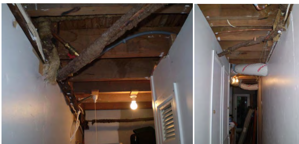
Photo of accessible area that would benefit from underfloor insulation. This is directly under the hallway, bathroom entry and kitchen.
