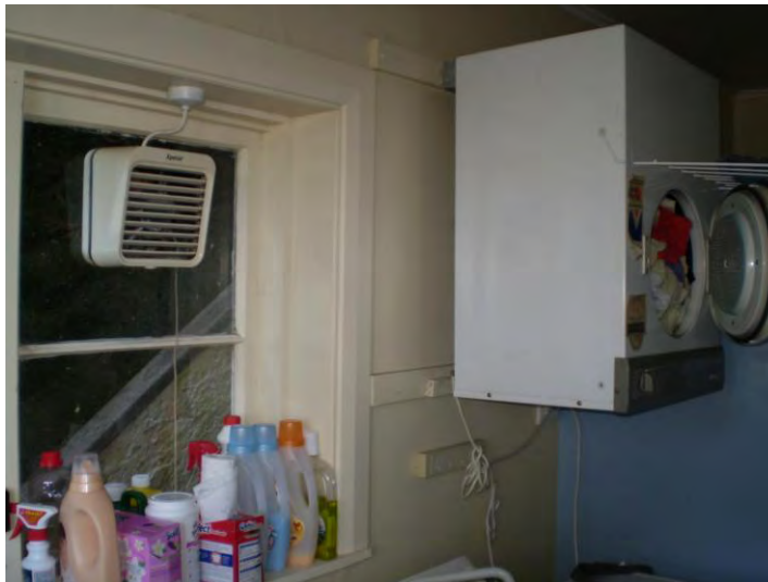
Photo showing the laundry room/ensuite directly off the ground floor bedroom. The dryer and shower should be vented to the outside. This is adding to internal moisture content.
