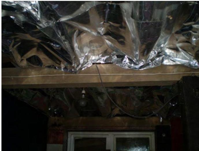
Photo of the foil layer directly below the master bedroom. The installed foil is not effective and needs to be replaced. The foil should be fit flat across the floor joists with no draping.
