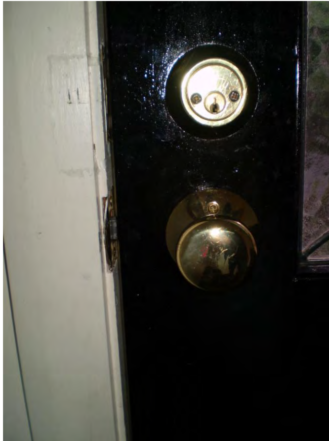
Photo of ground floor rear door which has a significant gap particularly around the door catch and does not close tightly.
