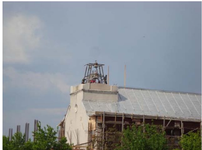
May 10, 2009 – the demolition continues after the court order
