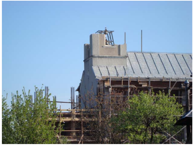
May 1, 2009 – the greek-catholic church during the demolition
