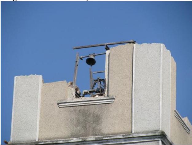
May 1, 2009 – the greek-catholic church during the demolition
