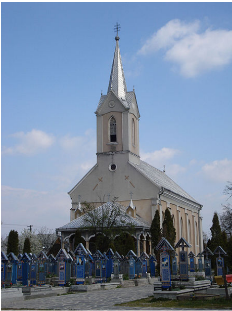
the greek-catholic church prior to demolition
