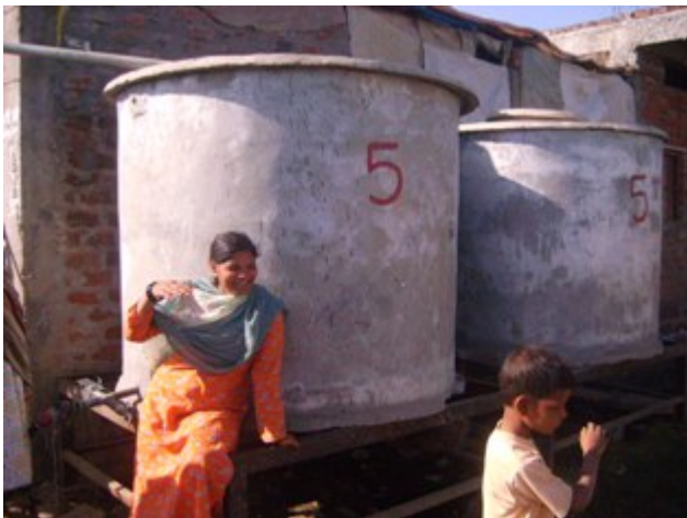
Figure 13: Concrete water tanks are smaller than the plastic tanks
