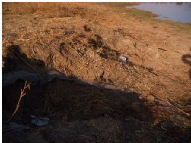
Figure 35: A thin polyethylene plastic layer, covered with soil, was supposed to prevent leaching of the pond water into the groundwater
