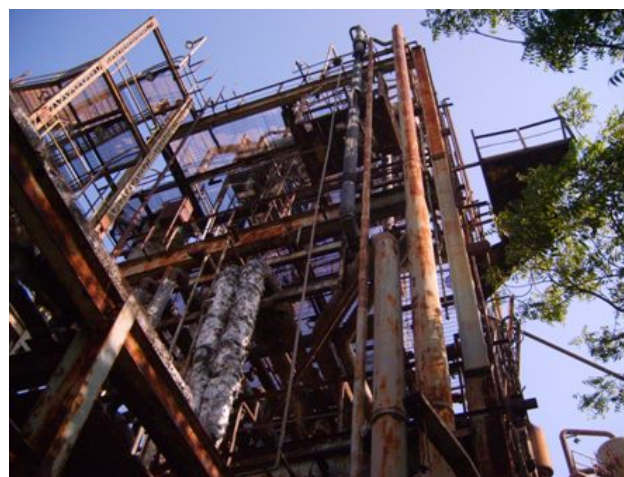
Figure 38: Close-up of a rusty formulation tower of the UCIL plant
