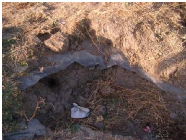
Figure 36: Disruption of the plastic layer on the dam of the SEP
