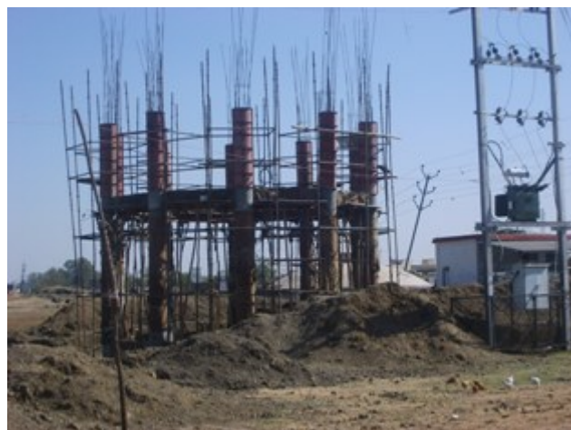
Figure 24: Construction of an overhead water storage tank, with a capacity of 1'000'000 litres, in addition to the existing ground storage tank, for the pumping station,.
