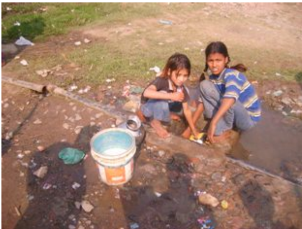
Figure 31: Ruptured pipe in Shri Ram Nagar
