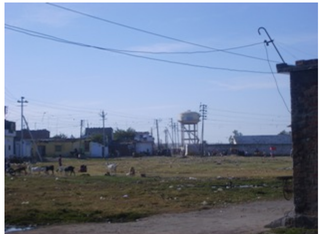
Figure 32: Overhead water storage tank in Arif Nagar which used to supply parts of the community with water by a pipe network. The network is broken and hence New Arif Nagar does not get water from the tank
