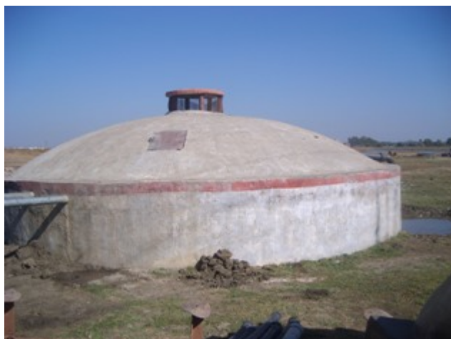
Figure 23: A so-called sub-tank (ground storage tank) at the pumping station in Blue Moon Colony with a capacity of 400'000 litres. The tank was built in 2005.
