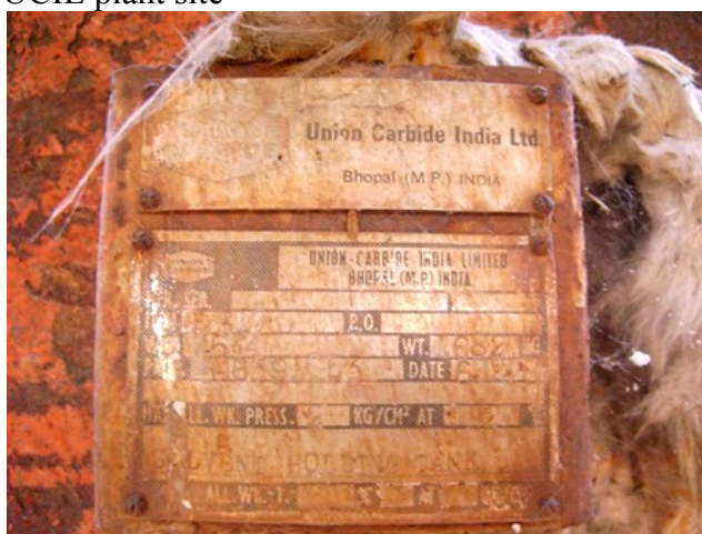
Figure 39: A badge from a former solvent holding tank
