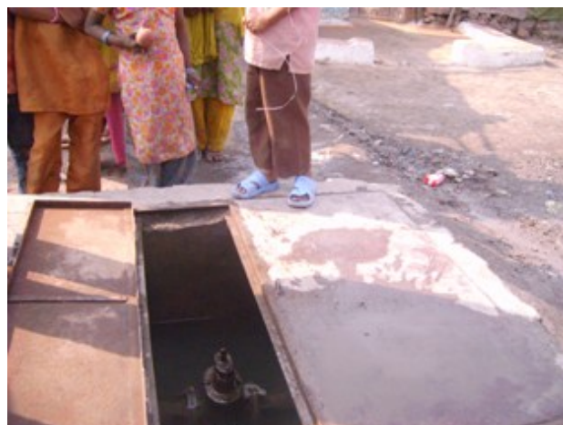
Figure 18: Individual switch of the water pipe network in Annu Nagar, which supplies the tanks individually with water from Rasla Khedi
