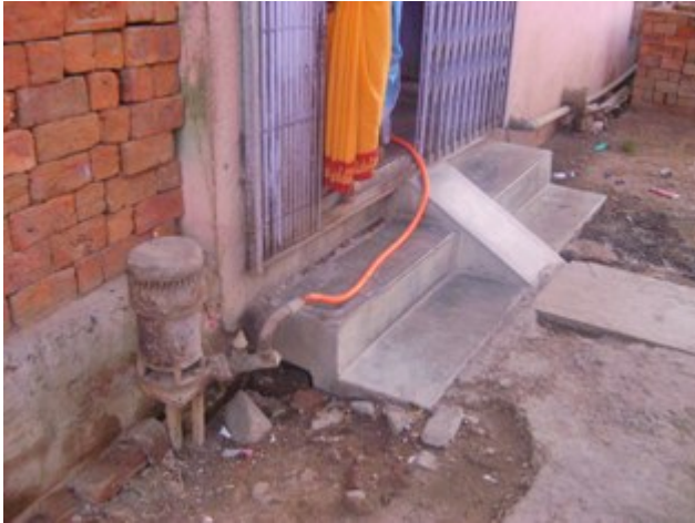
Figure 7: Bore well in front of a house
