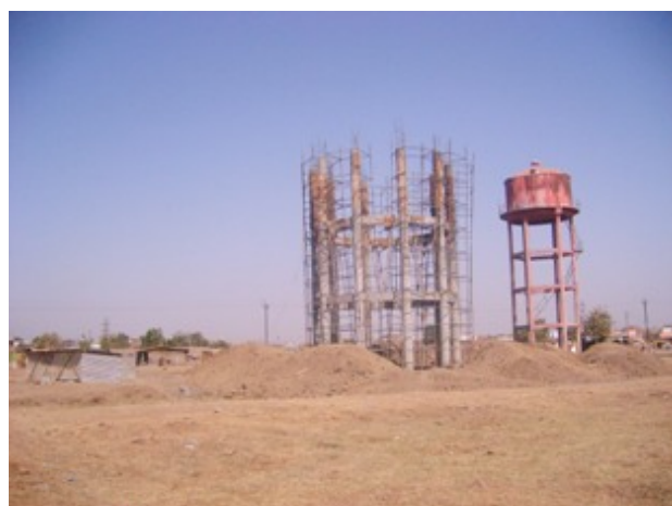
Figure 20: Old overhead storage tank (right) and construction of a large overhead tank (left) in Chandbaadi
