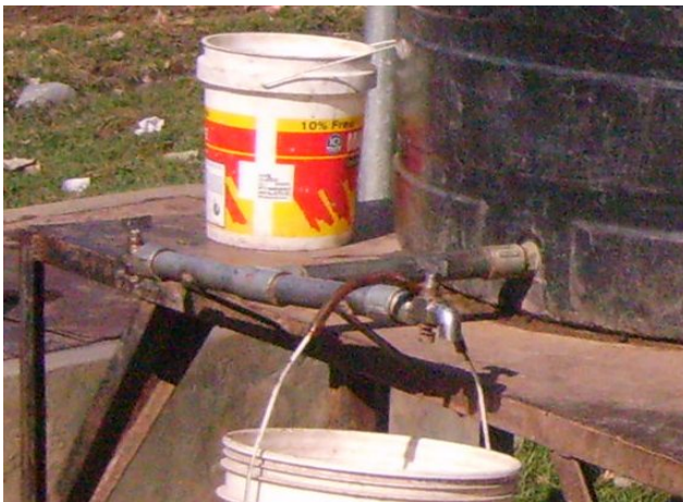
Figure 27: Water tap, the most vulnerable part of a tank because it tends to easily break
