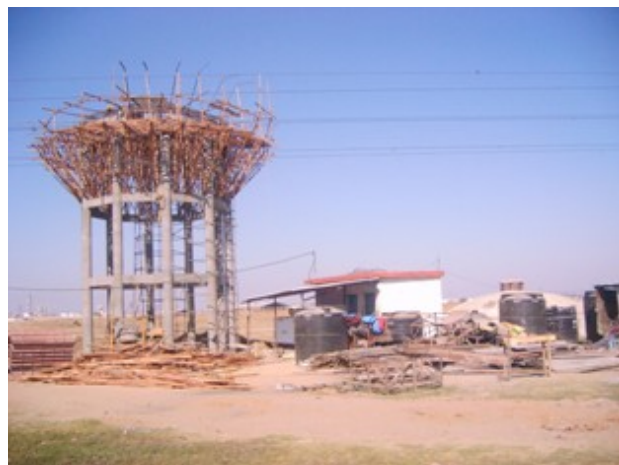
Figure 22: Construction of overhead water storage tank at Blue Moon pumping station.
