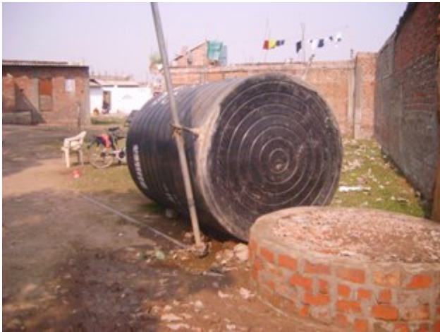
Figure 29: Broken tank in Shri Ram Nagar
