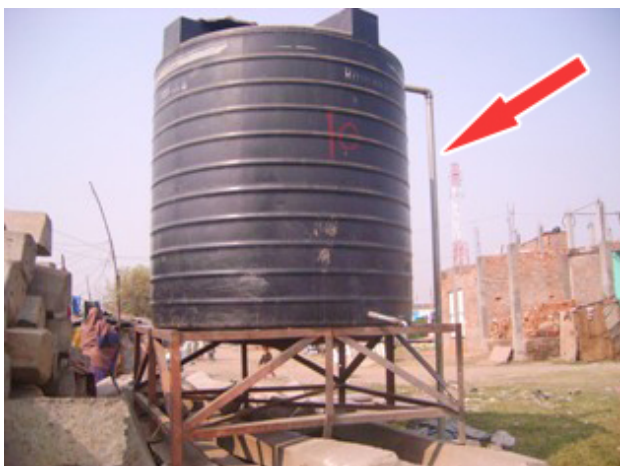
Figure 17: Water pipe marked with red arrow
