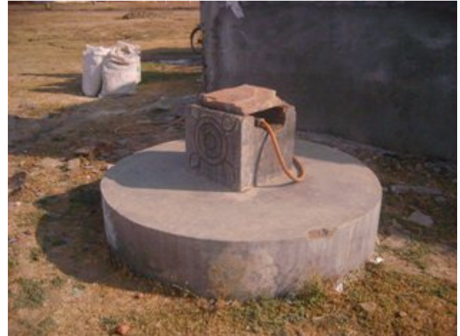
Figure 8: Bore well sheathed in a concrete wall
