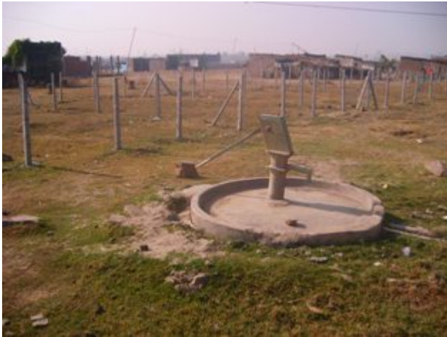
Figure 2: Public hand pump, out of commission
