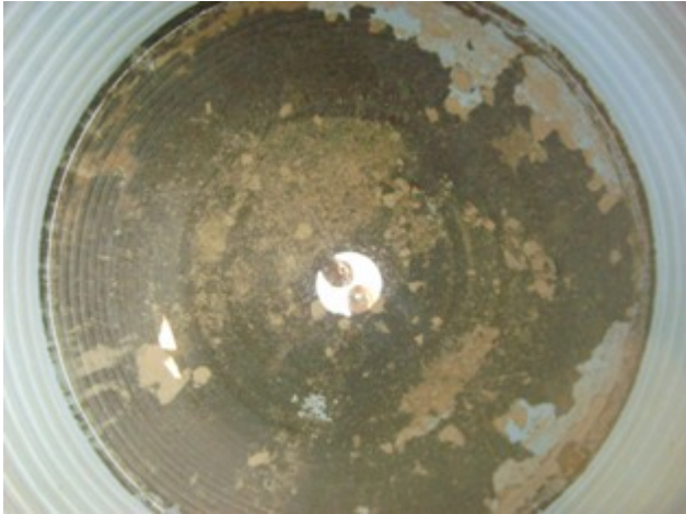
Figure 25: Algae and dirt inside a water tank which has not been refilled on a regular basis. The tank is located in Blue Moon Colony.
