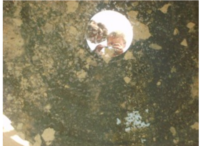
Figure 26: Bottom of the water tank from Fig. 26
