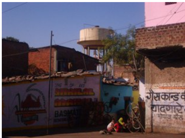
Figure 21: Overhead tank in Jaiprakash (J.P.) Nagar
