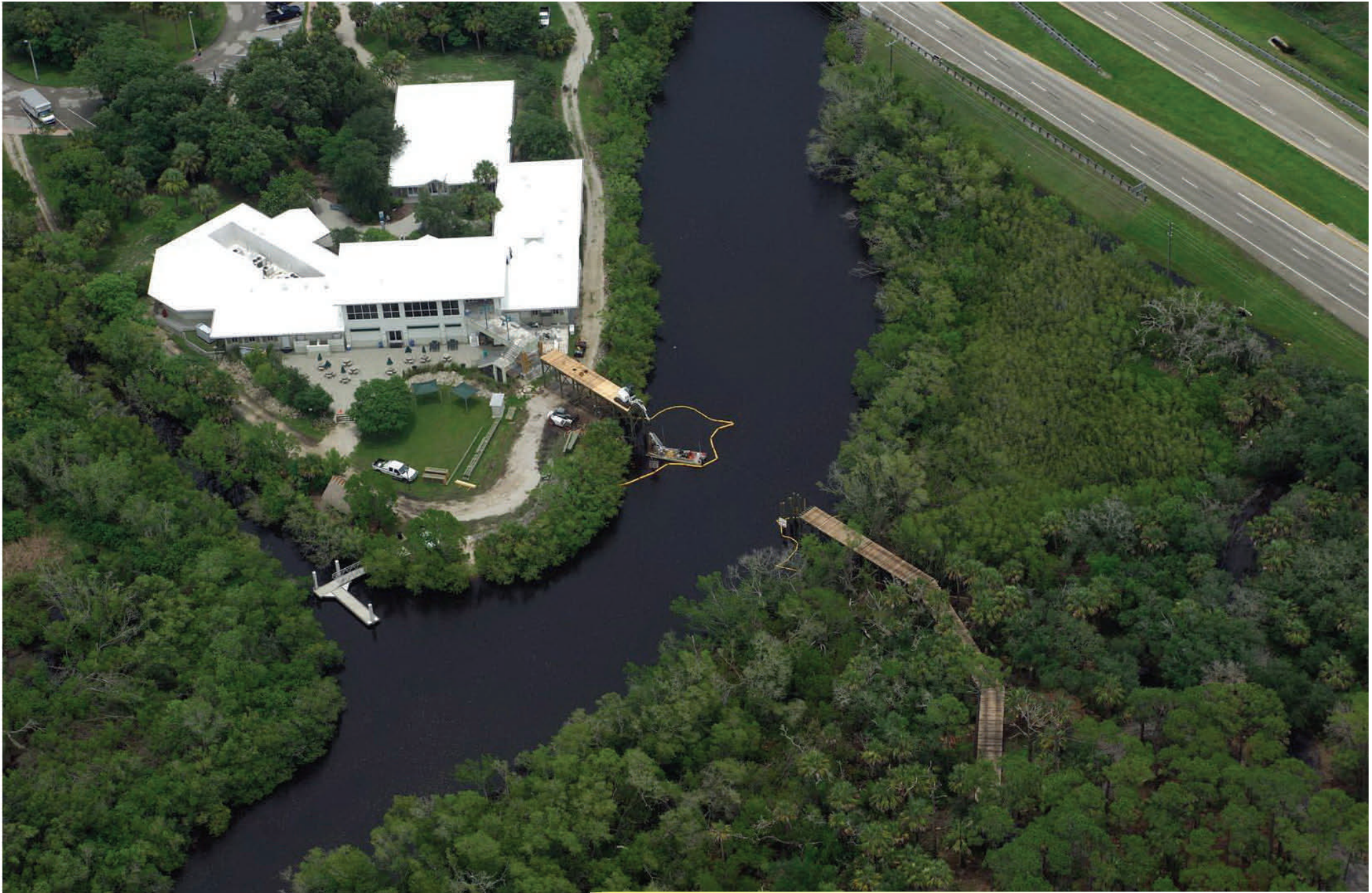
North side connector to 2nd floor observation deck. Construction being performed from barge in the waterway and excavator on the bridge.
