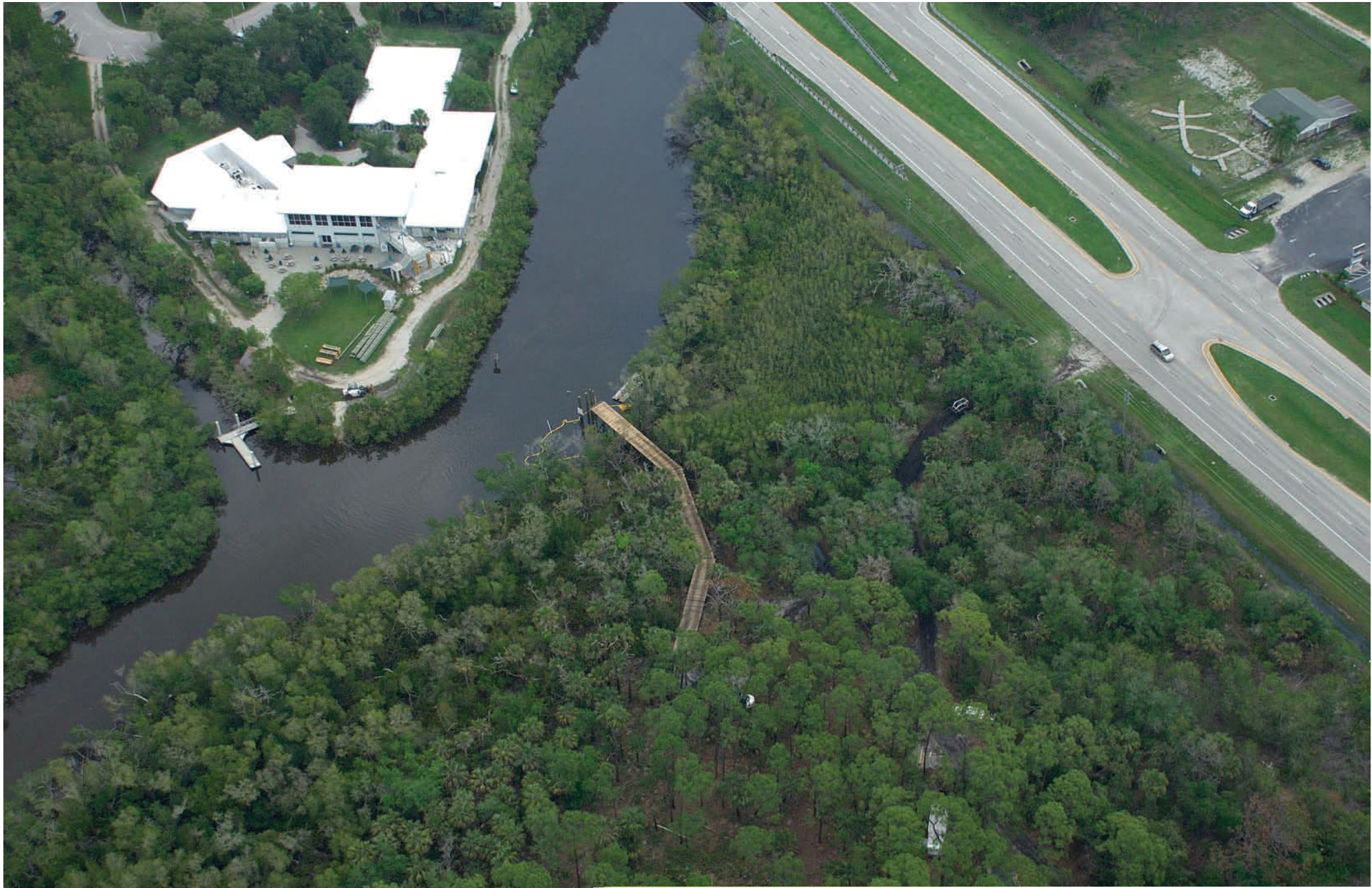
Birdseye view of completed Southside approach. Abutments being prepared for free-span section.
