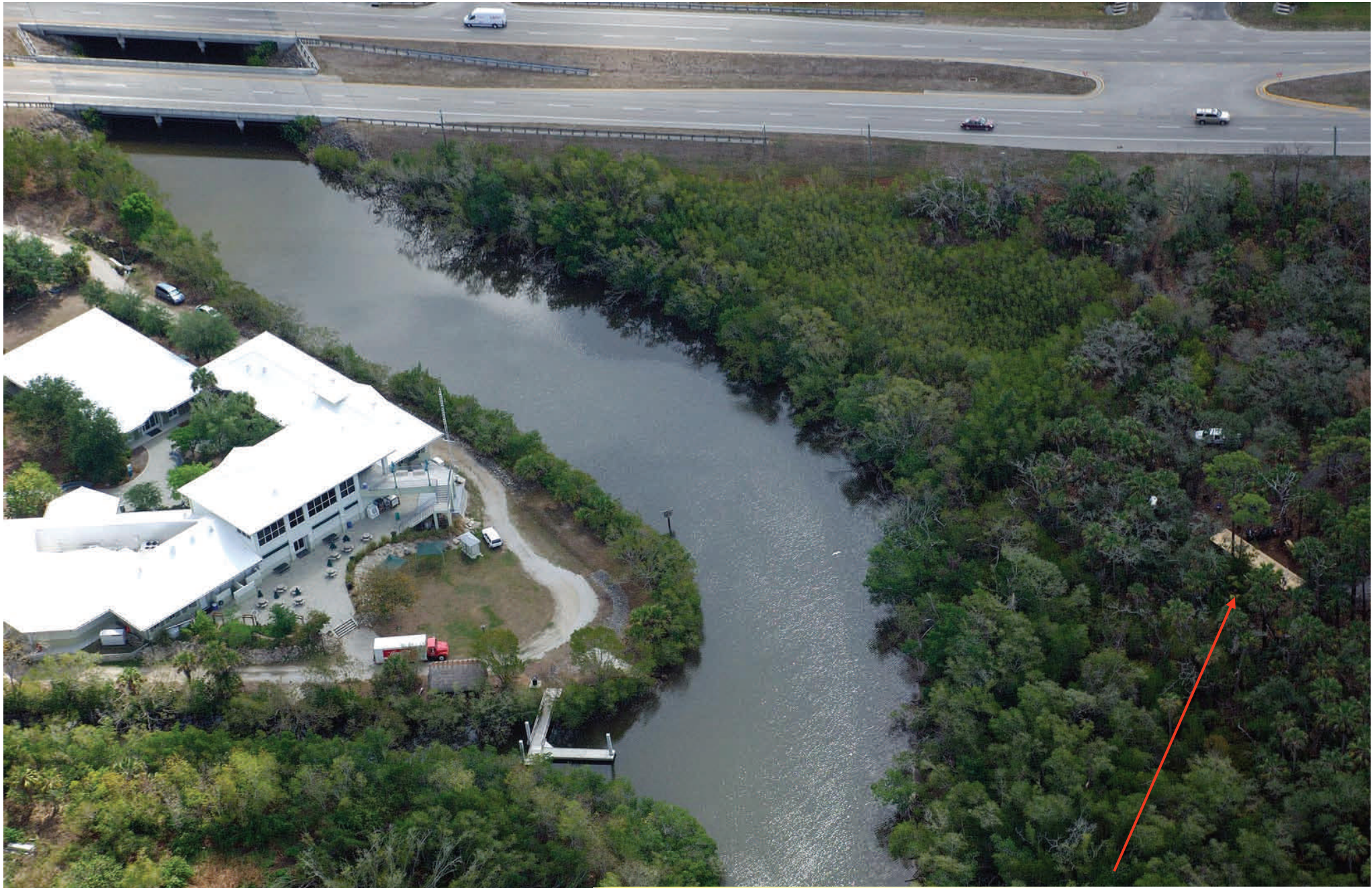
Project location with some boardwalk started on initial approach on Southside.
