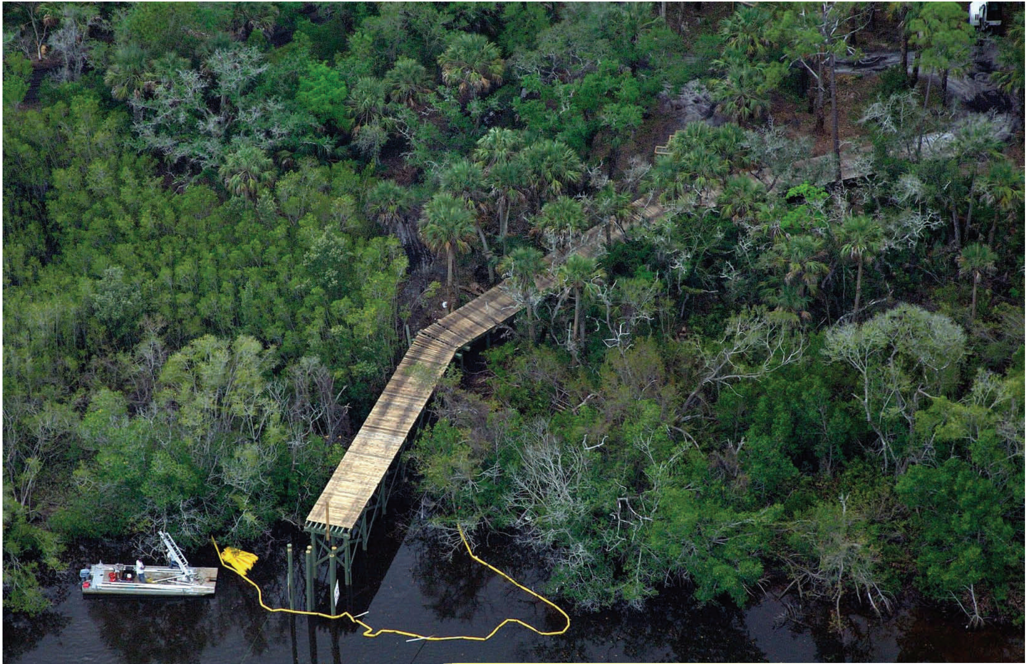
Construction coming from south side of Henderson Creek. Barge in place for pile setting and structural framing process. Temporary timber decking for top down construction method. Fiberglass reinforced — plastic decking installed after removal of heavy equipment from bridge.
