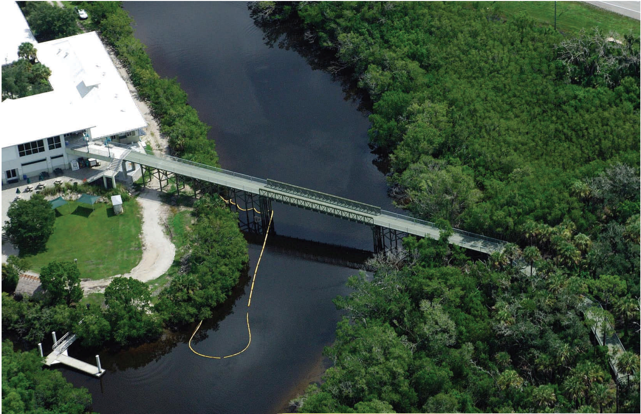
Completed project. Pedestrian bridge begins on the 2nd floor at the Learning Center, continues across Henderson Creek and into Rookery Bay Estuarine National Preserve where visitors can experience historical sites and the natural habitats throughout the estuarine.
