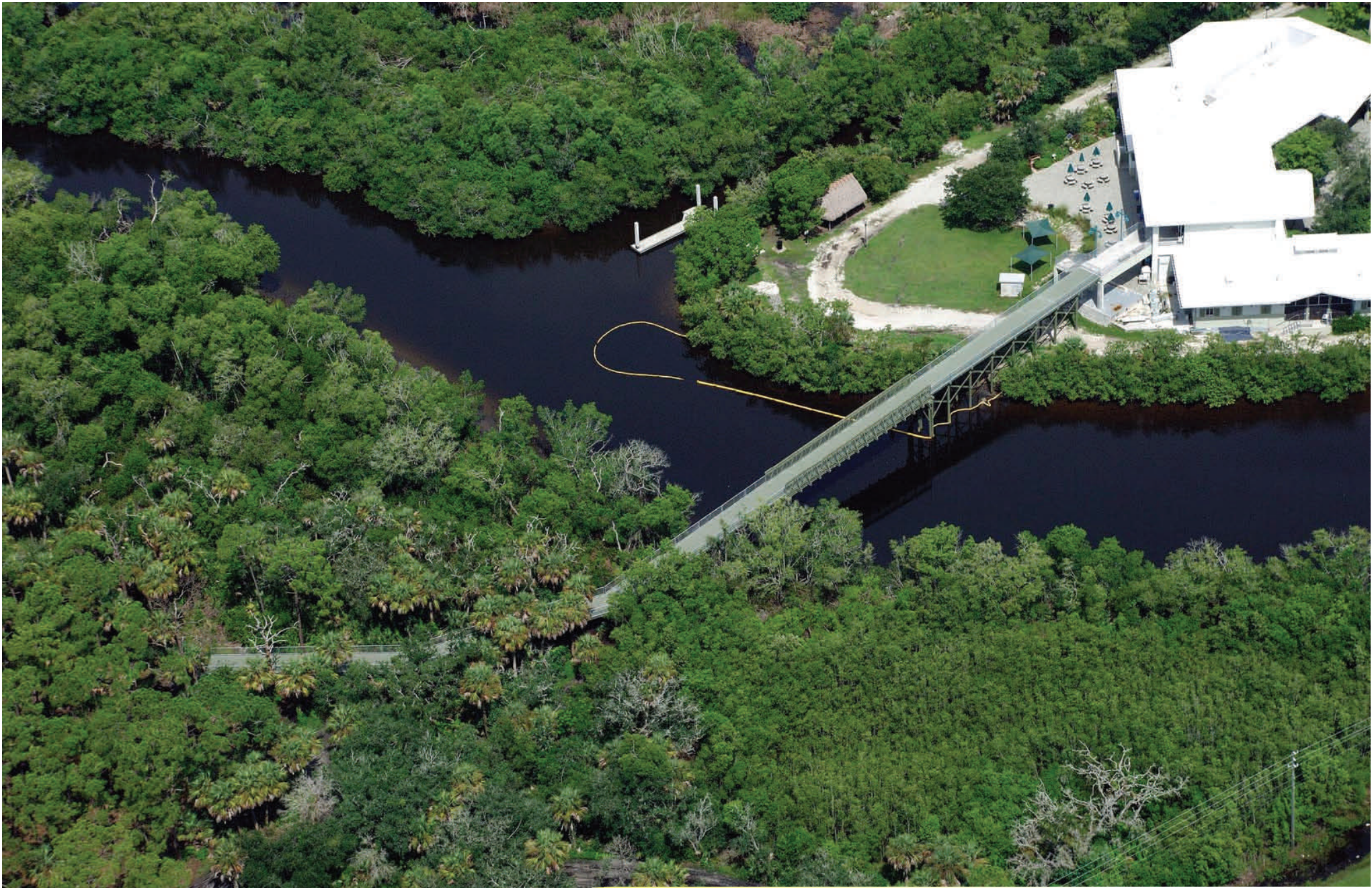
Project completion. Permanent fiberglass reinforced plastic deck panels installed. View from south side of project.
