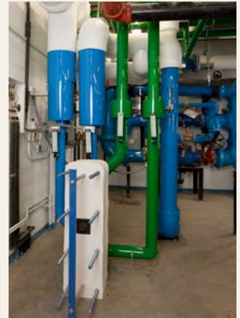
Figure 4 Plate frame heat exchanger near vacuum pump No. 1
