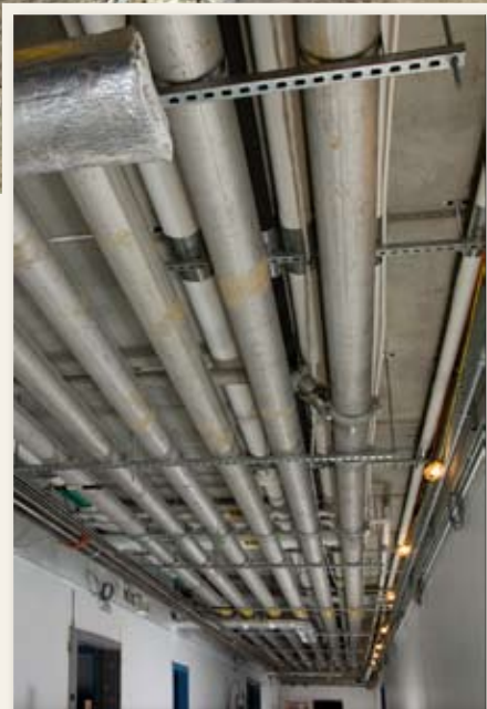
Figure 2 Overhead vacuum waste piping
