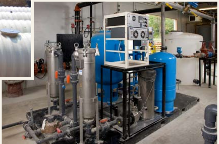
Figure 7 Rainwater harvesting system
