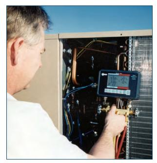
Don't have a refrigerant manifold gauge? Consider a digital refrigerant system analyzer. Automatic subcooling and superheat readings make it easier to determine the proper refrigerant charge.
