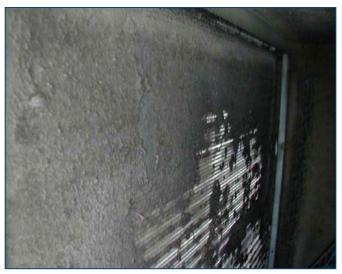
Filthy Cooling Coils Restricting Airflow and Cooling Effectiveness. Closer inspection revealed missing air filters.
