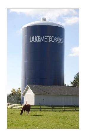
The exterior of the Metro Farms standpipe in Kirtland, OH was coated with Series 740 UVX because of its resistance to abrasion and exterior weathering.
