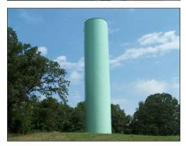
Series 27WB was chosen for the Trappist, Kentucky water tank because it serves as an excellent tie coat on previously painted surfaces and forms a very hard film when cured.
