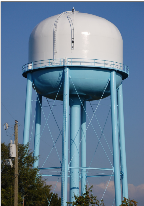
The exterior of the 500,000-Gallon Elevated Water Tank in Perry, GA was coated with Series 740 UVX because of its low-VOC content and exterior weathering properties.
