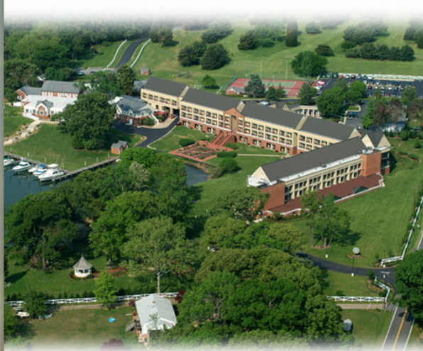
William W. Winpisinger Education and Technology Center at Placid Harbor, Maryland.
