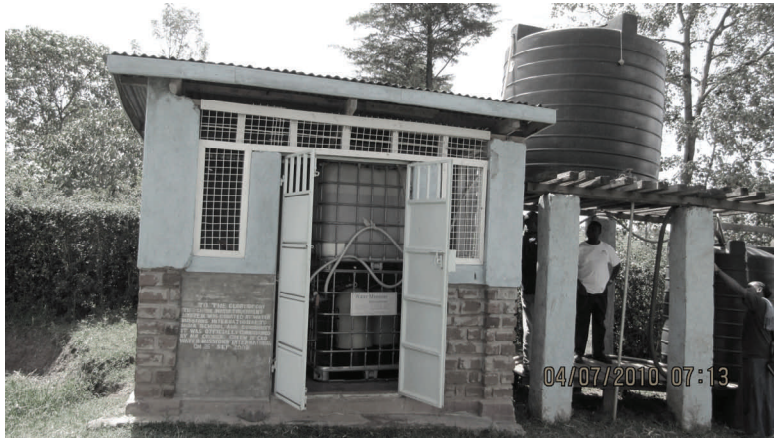
A completed filtration system installed by Water Missions in another Kenyan village
