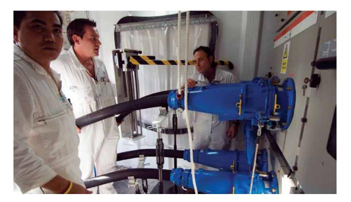
A new alternative that is emerging within the cruise ship industry is the ability to "plug in" while in port, connecting the ship to shore-side power and shutting down its own engines, also known as "cold ironing."
