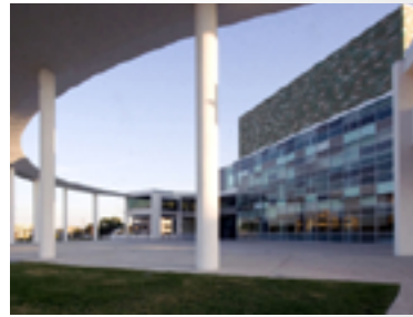
Aluminum panels from the original structure's dome added color to the Long Center's facade.
