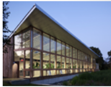
A living building, the Omega Center incorporates reclaimed Cypress as part of its commitment to tread lightly on the earth.
