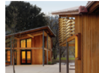
Portola Valley Town Center. Reclaimed Yellow Cedar was used to create sunscreen louvers. The buildings are clad in reclaimed redwood.
