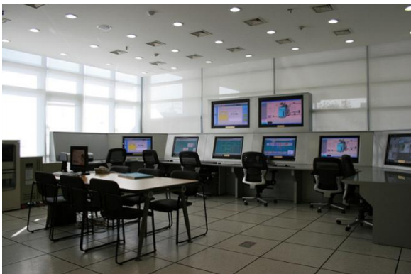
Monitoring Room - AnC Bio Headquarters - Korea
