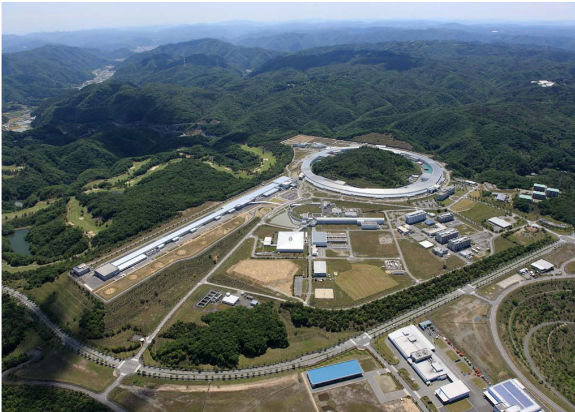
Figure 1: Aerial photo of the SPring -8 campus. The long structure extending diagonally to the bottom-left is the X-ray Free-Electron Laser (XFEL). To its right is the storage ring of the SPring-8 synchrotron.
