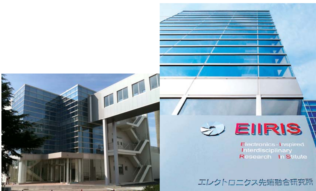
Fig.2: Photographs of the EIRIS building
