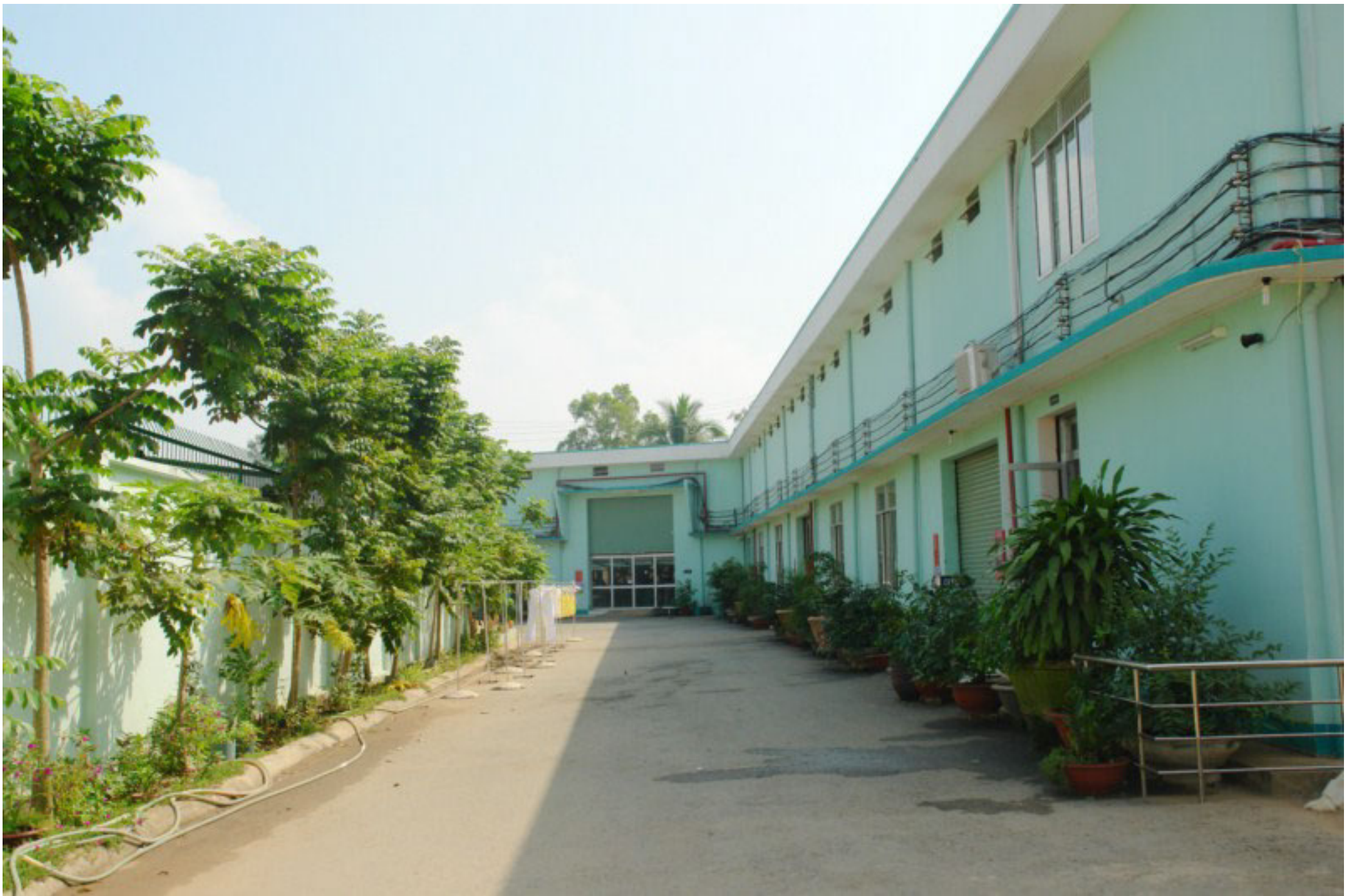
03 Factory internal road - from main gate
