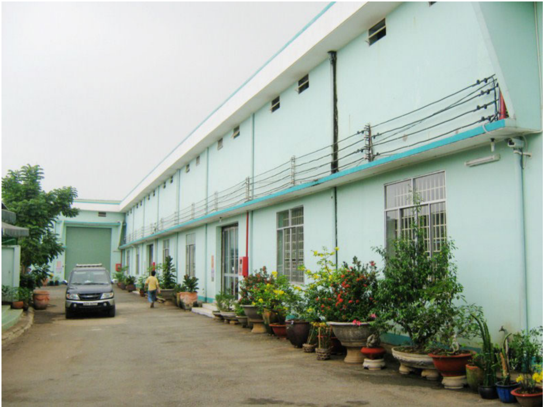
04 Fatory internal road - to fabric warehouse
