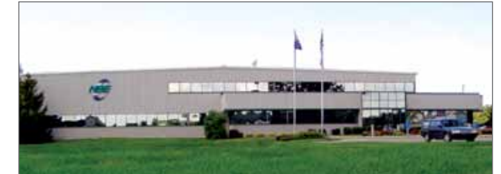
NBE operations cover over 70,000 square feet and include manufacturing, R&D, and UL listed controls construction.
