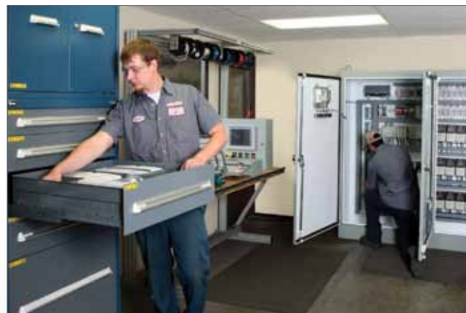
All NBE controls are custom-built in a dedicated, on-site UL certified panel build facility. NBE panel configurations include 508 or Class I, Division 1 and 2, Groups A-D, F and G, NEMA 12 enclosures with Type X purge.
