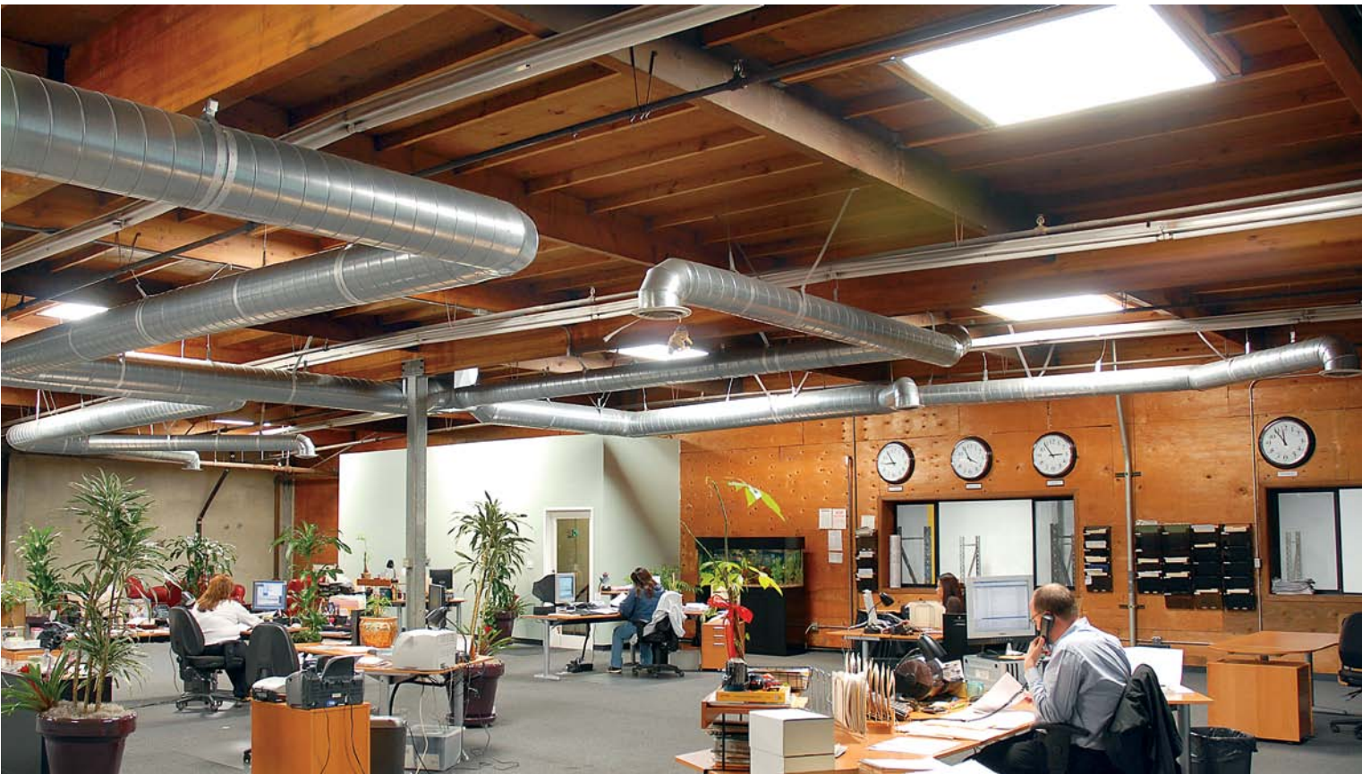
A-1 Cold Storage near the LAX airport has no out-facing windows yet this office is daylit and all fluorescents are off!
