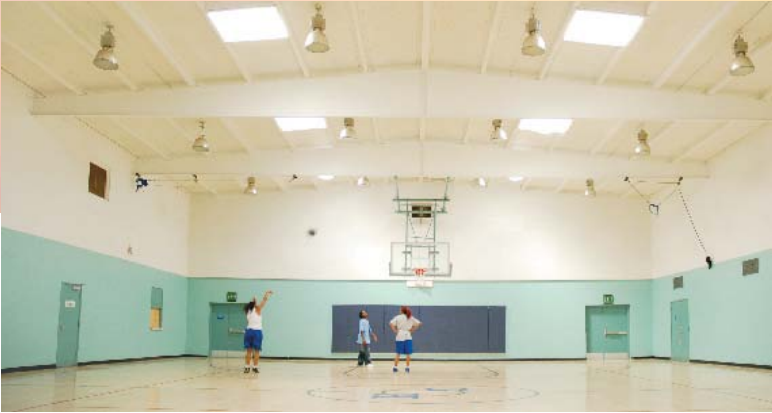
This City of San Diego Community Center is lit entirely by Advanced Daylighting. The artificial lighting is off!
