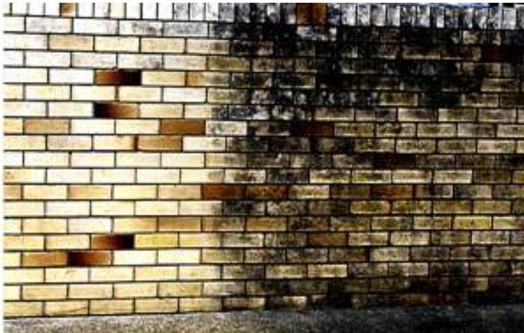
Brick Wall Before and After Application Wet & Forget
