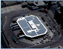
Otay Mesa Customhouse- This eight sided building located near San Diego at the Mexican Border was reroofed by BEST using a Weatherweld Roofing System. Weatherweld is a cold process sprayed in place system which results in a seamless, monolithic and waterproof roof. After the roof installation, solar BIPV was installed providing supplemental electric power to the facility.
