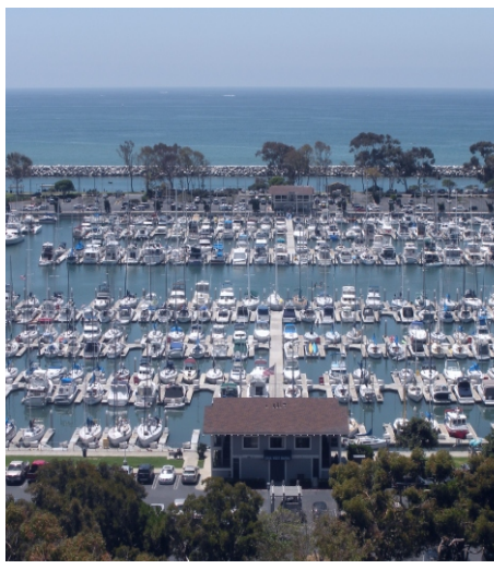
The Dana Point Harbor, a modern Marina on the Pacific Coast.
