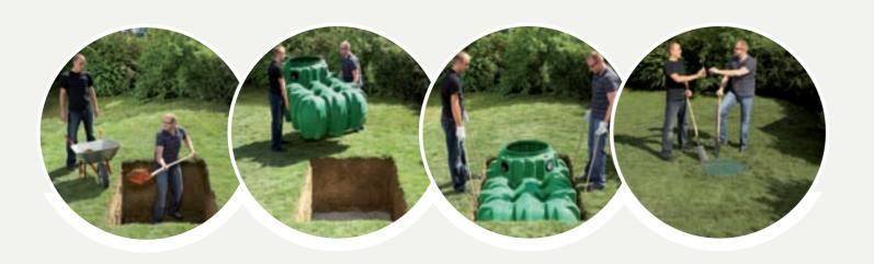
75 % less digging compared with a concrete cistern. Save more than 100 wheelbarrow loads of soil!
