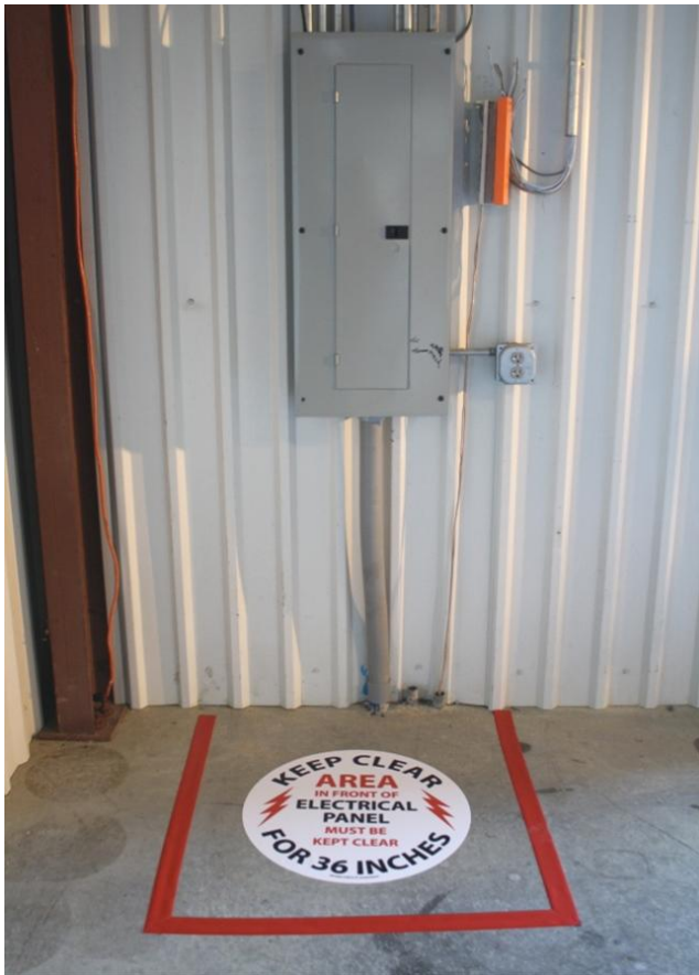
Electrical panel floor marking kits help facilities comply with OSHA regulation 1910.303 which requires the area around electrical panels to be kept clear for 36 inches.
