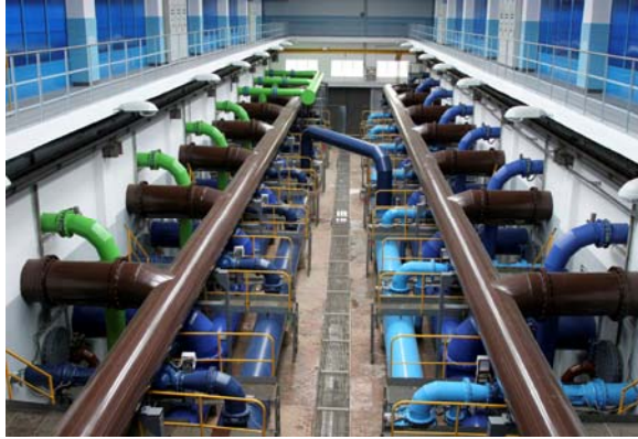
Inside a WWTP
