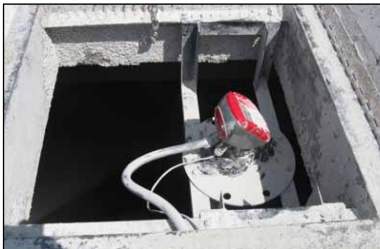
A dusty application in an ethanol plant.
