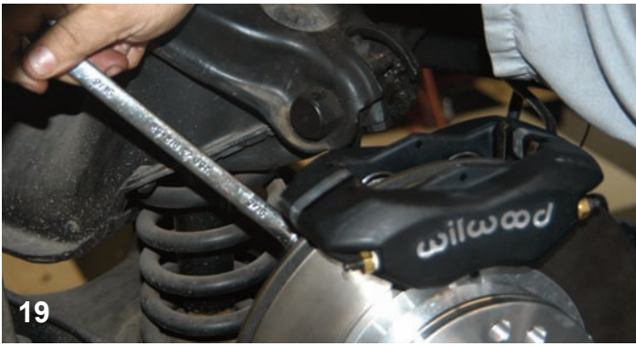
After the pads were installed, the caliper bolts were tightened. Tony made sure the caliper was centered over the rotor, and after it was, the bolts were coated with Loctite 271 and were tightened to 77 ft-lbs.
