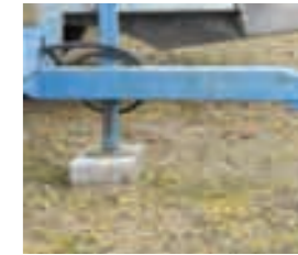
Porous parking area
