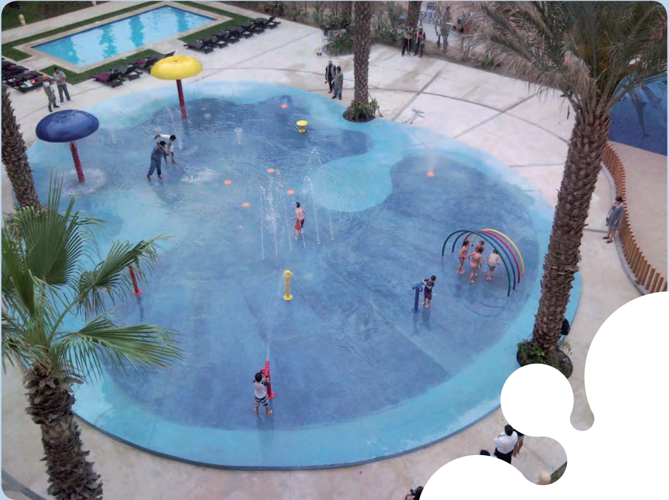
Barcelo Los Cabos Splashpad® in the final stages of installation
