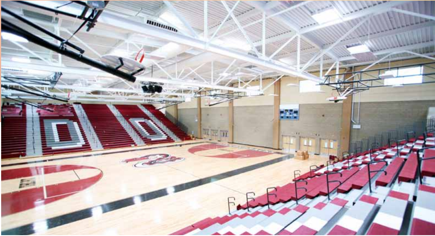
This High School Gymnasium in Las Vegas, NV is lit entirely by Ciralight SunTrackers. The electrical lighting is off!
