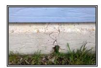
Cracks that are more than an 8<sup>th</sup> of an inch wide usually mean that the foundation has been bent. This may be a sign of foundation problems. It may be time for foundation repairs.
