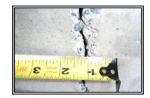
During foundation repairs, when foundations are lifted, cracks do not always close. Unlike fitting a cracked plate back together, the foundation will often not close. Foundation cracks are often held open by pebbles or pieces of concrete. In other cases the sides may have shifted just enough to prevent the crack from lining up perfectly.
