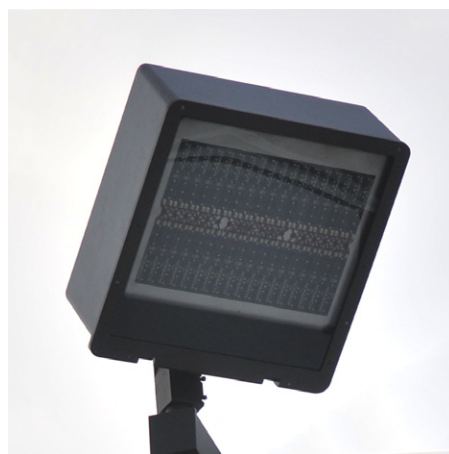
A Noribachi light engine, constructed of modular lightboards, visible inside a fixture.
