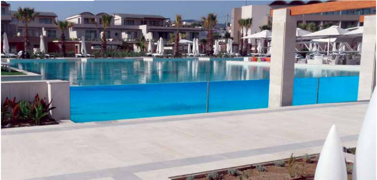
The sealant joints between the panels in this pool allow for larger views directly into the water while using multiple smaller panels. The sealant minimizes the amount of obstructed views while maximizing overall window size.
