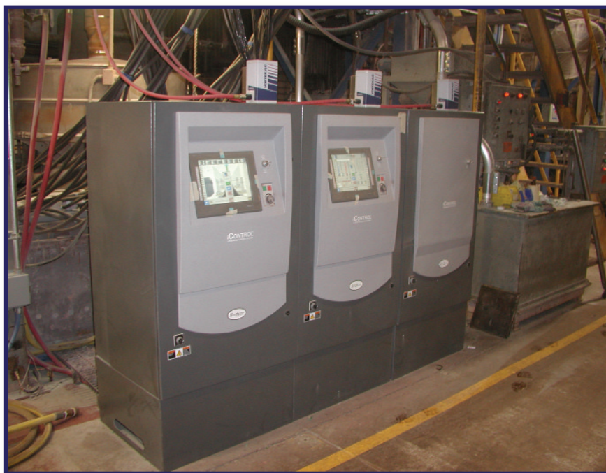
The compact size of the Vortex A/C units proved to be an important advantage when EB Pipe Coating purchased a new system that required three control panels to get 48 powder coating guns. The panels needed to be pushed up next to each other, which couldn't be done with conventional air conditioners mounted on the side of each panel
