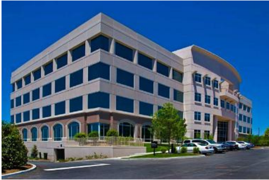
PICA Building – Franklin, TN
