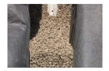
After the pipe is laid, the trench is filled with gravel to within a few inches of the surface.
