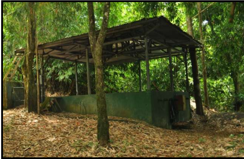
Laundry Grey Water Plant
