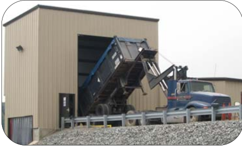
Truck-to-Rail transfer of contaminated soil.
